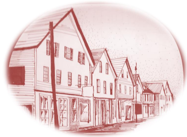
Water Street at King (from early 1980s)
